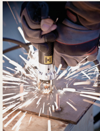
Welding studs to the rear of the Corten ribbon.
